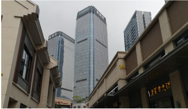
Figure 7: Zhuhai midtown consists of 2 grade-A office towers and retail shops
