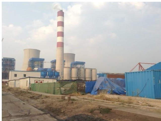
Figure 7: 4*330MW power plants
