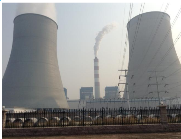
Figure 13: 4*330MW power plants
