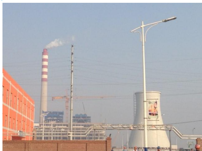
Figure 16: Power plants 2*60MV
