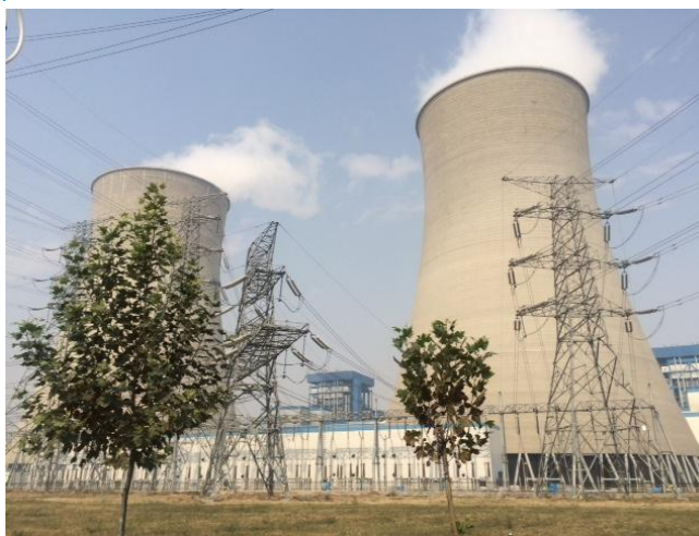
Figure 5: 4*330MW power plants
