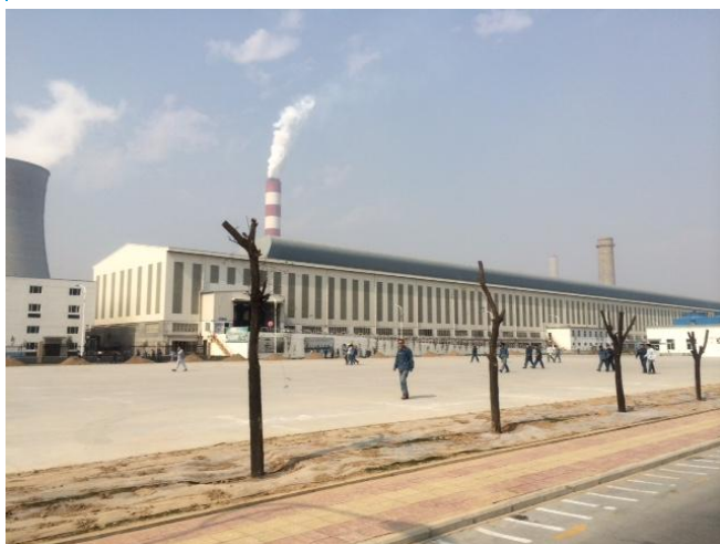
Figure 4: Aluminium production line in Huiming
