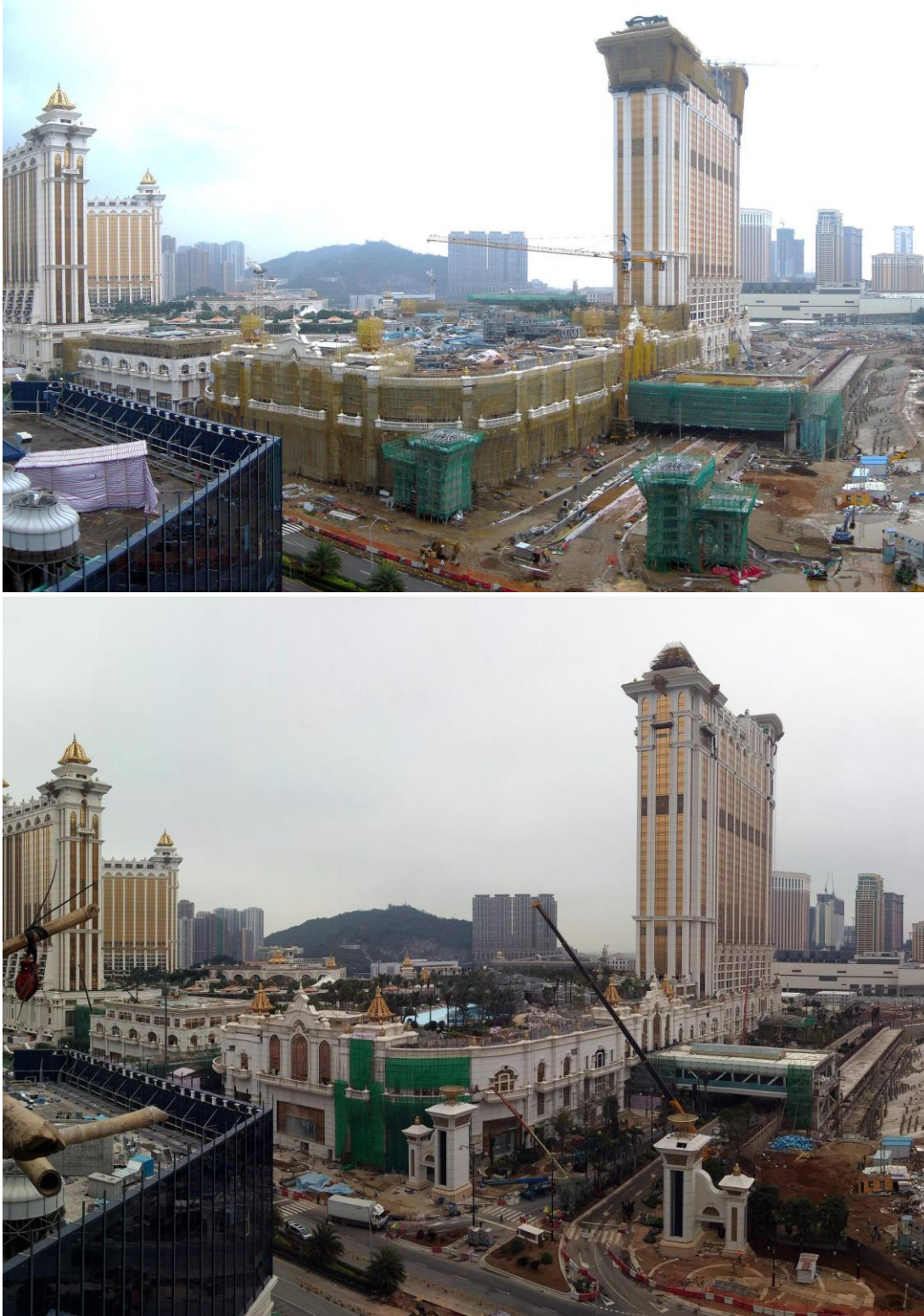
Figure 5: Galaxy Macau Phase 2 construction progress (November 2014 vs. March 2015)
