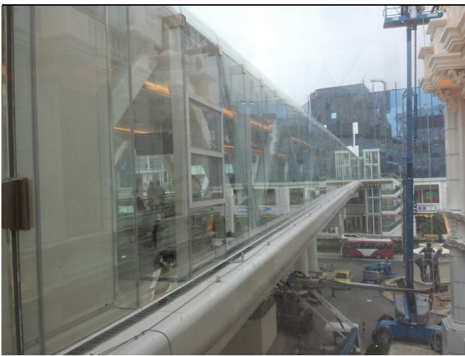
Figure 19: Footbridge linking phase 2 to Broadway
